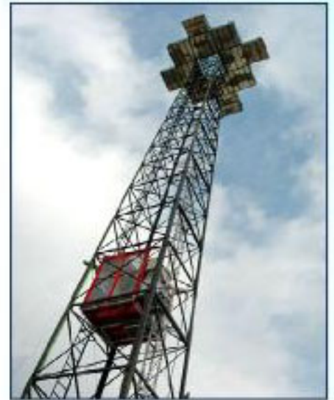
Elevator in transit
