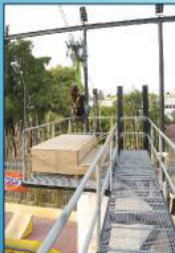
Elevated landing station
